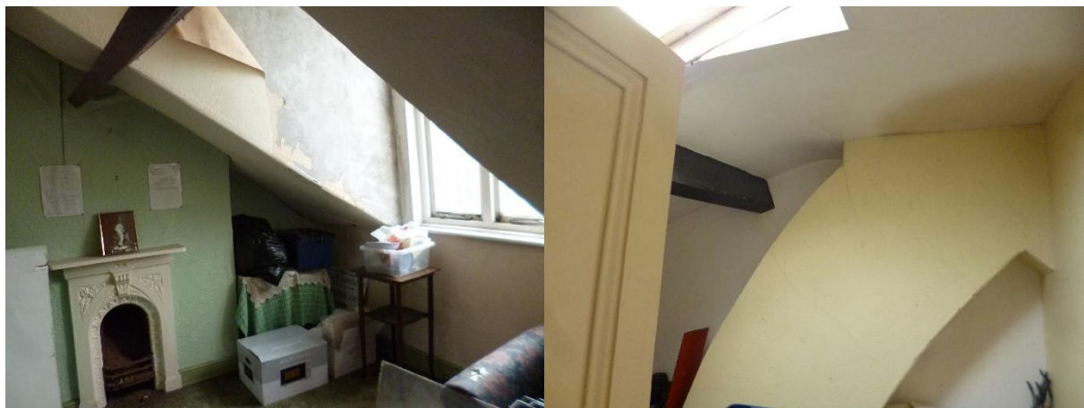
Fig.25: front attic room (left) and rear attic (right)
