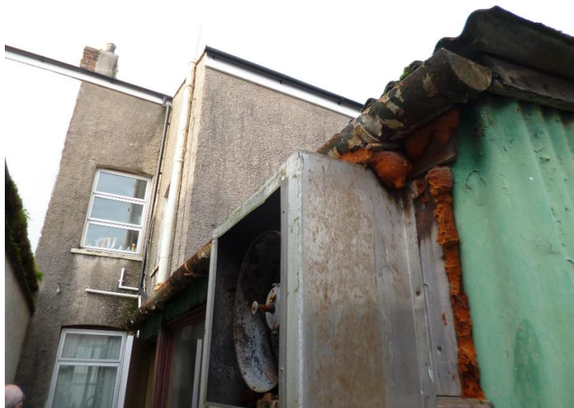
Fig.18: rear elevation, outshut and shed from the rear.
