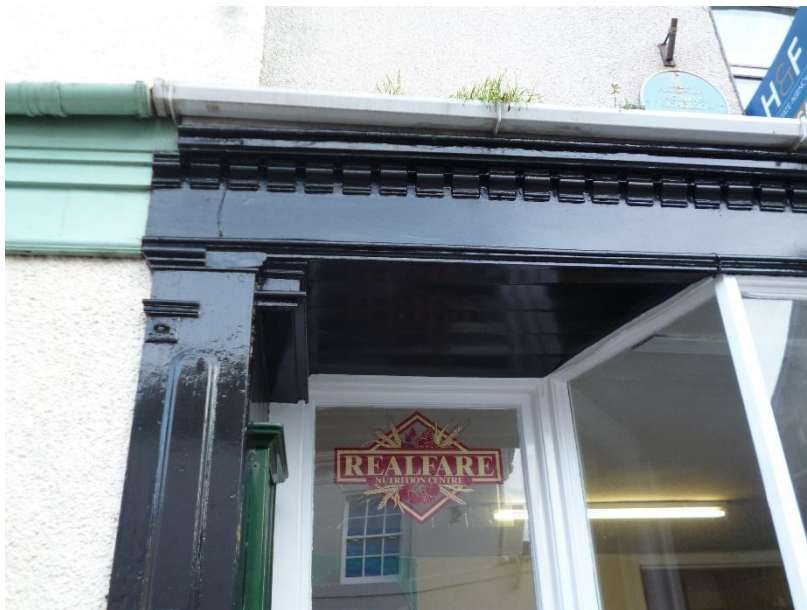
Fig.16: some original shop front details have survived
